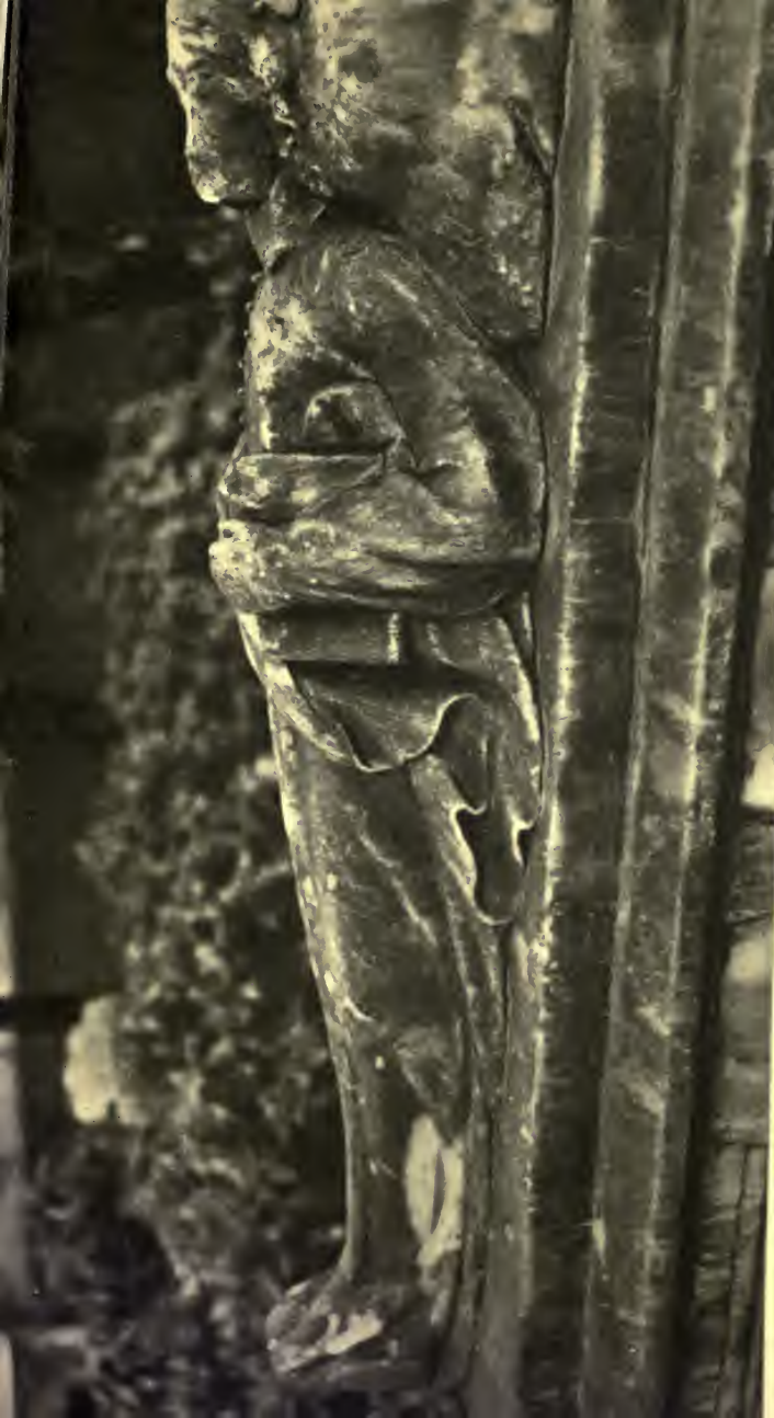
THE SHELL-DAMAGED EFFIGY OF JOHN BUNYAN IN BUNHILL FIELDS Executed by E. C. Papworth in 1861.
